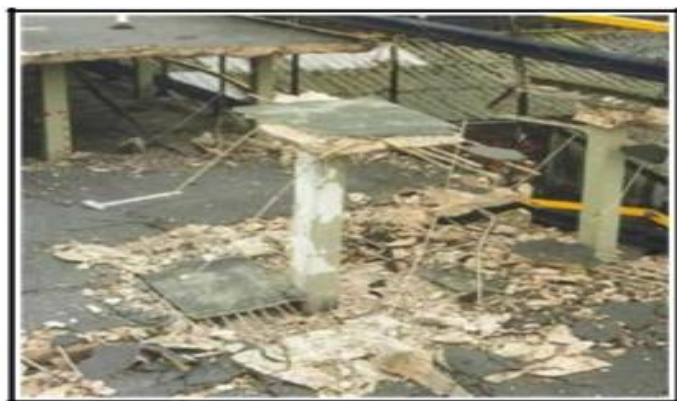
Fig6. Global collapse of the structure due to punching shear.
