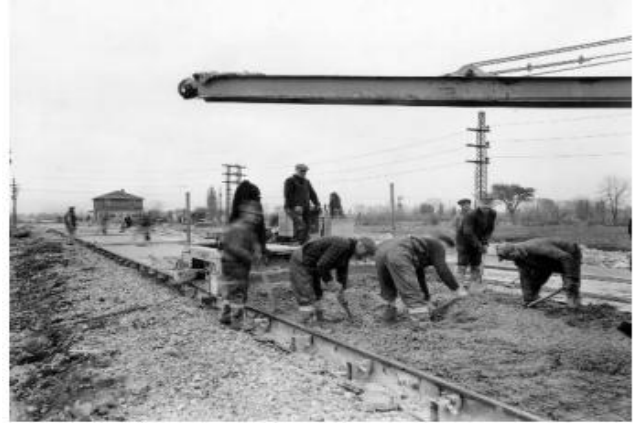
Fig.2. Early Concrete Pavement Construction In Québec.
